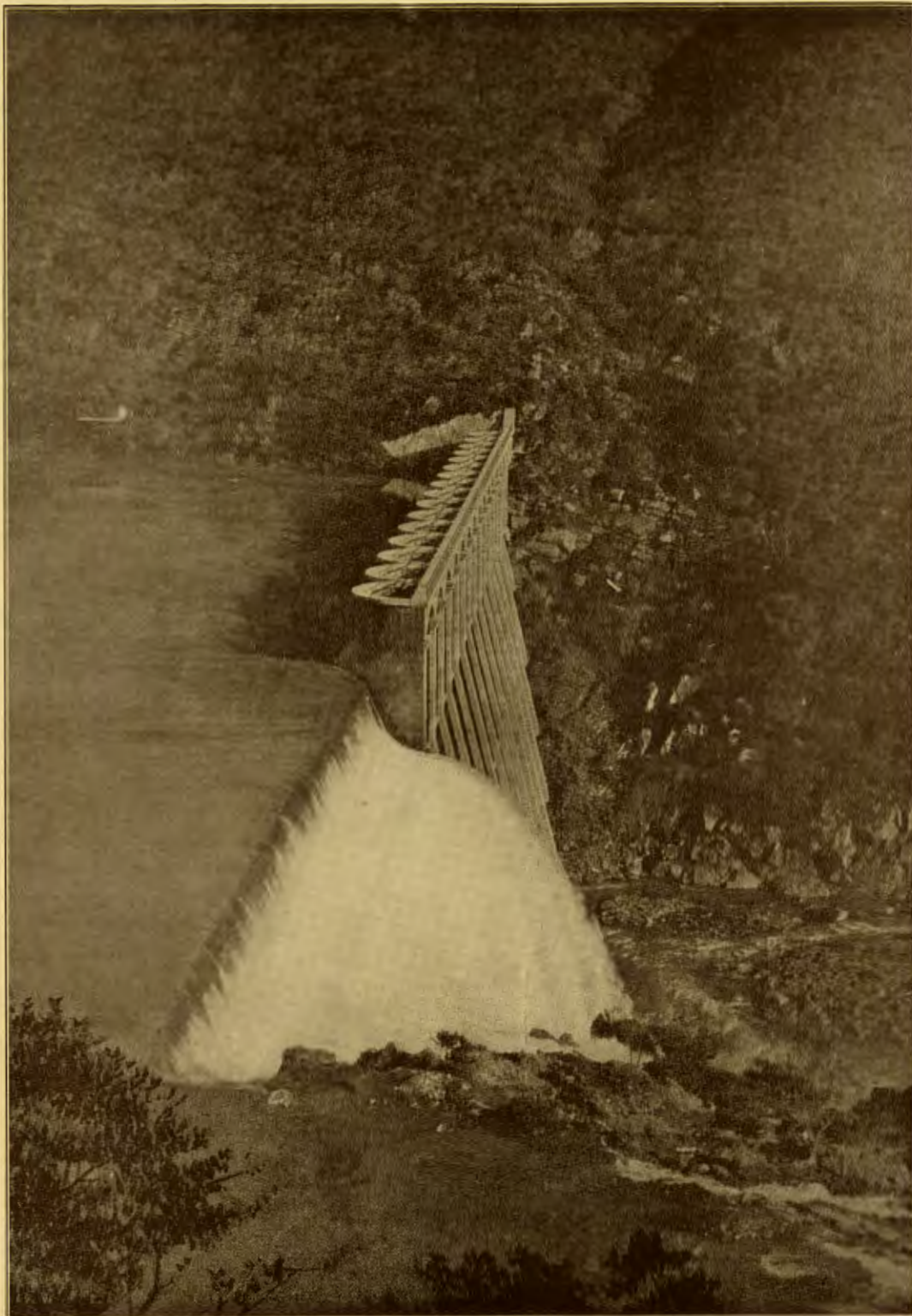
Lake Hodges Dam. 157 feet high; 750 feet wide.
