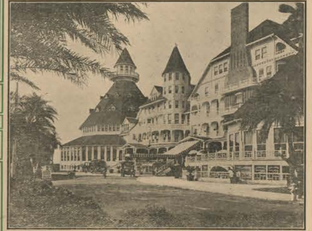
View of the Main Entrance
