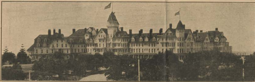
North View, Indicating the Immense Size of the Hotel
