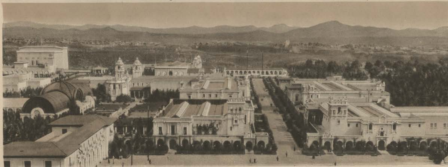
Looking East from Tower of the California Building.
