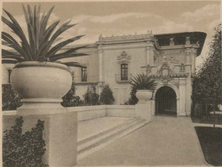
Vista of Commerce and Industries Building.
