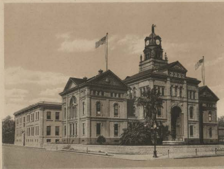
County Court House and Hall of Records.
