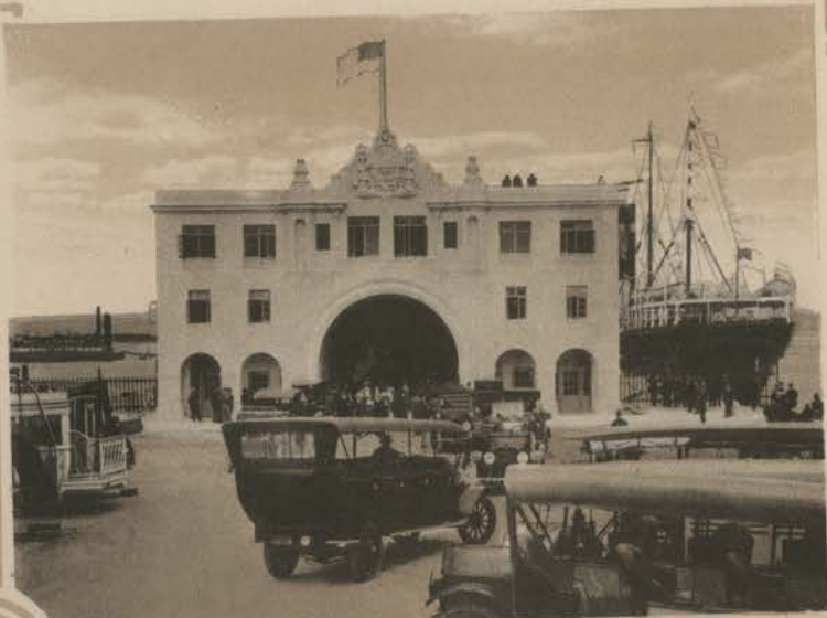
New Municipal Pier.
