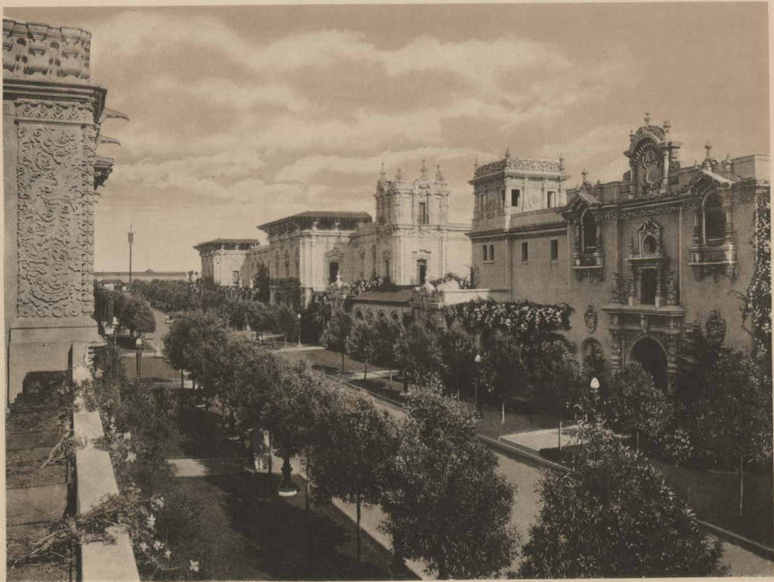
El Prado showing Commerce and Industries Building.
