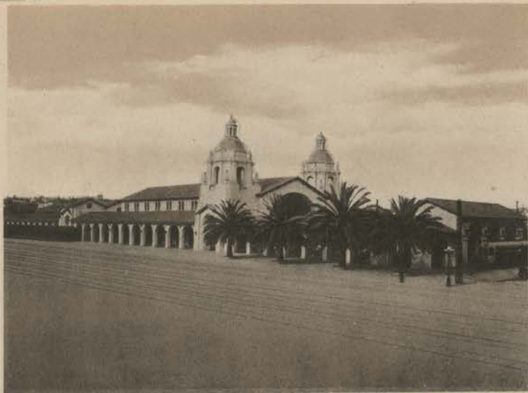
Santa Fe Railroad Depot.
