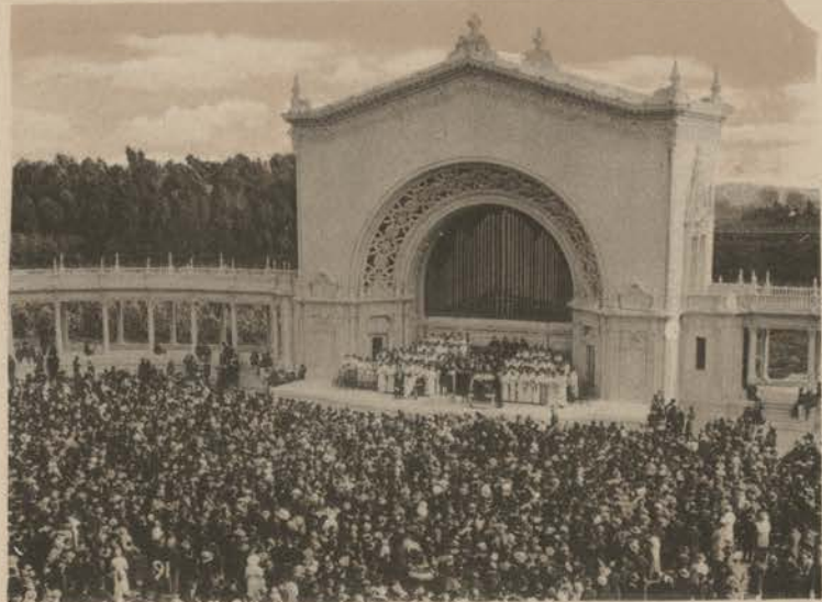
Spreckel's Pipe Organ.
