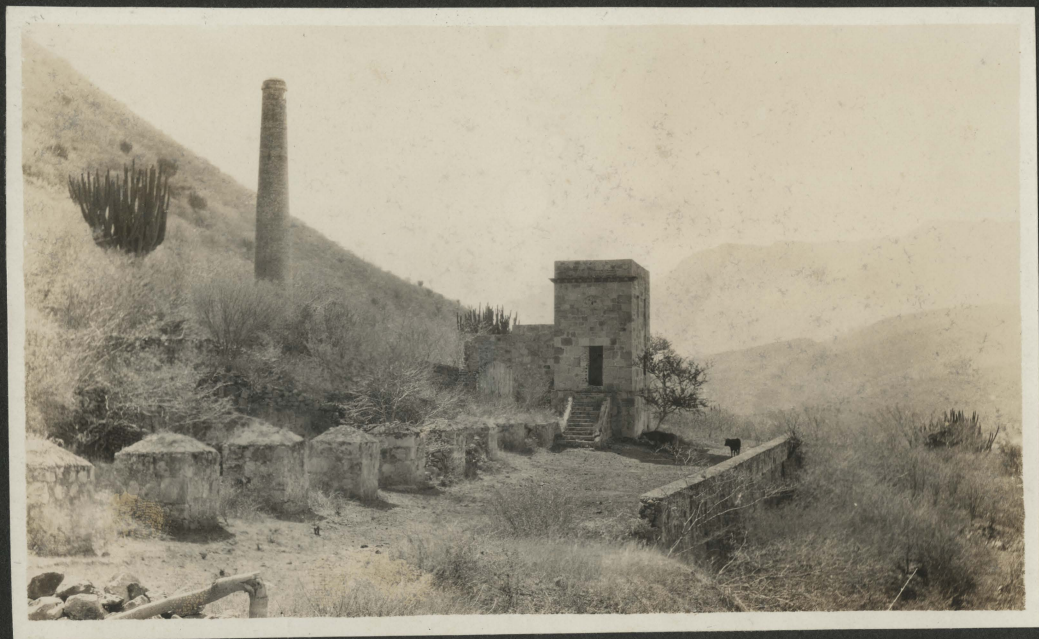
Balaños, Jal. - Dec. 1921 Old Santa Fe engine house viewed from the North, showing masonry supports for old Cornish pump "rods" (horizontal from engine house to shaft.)
