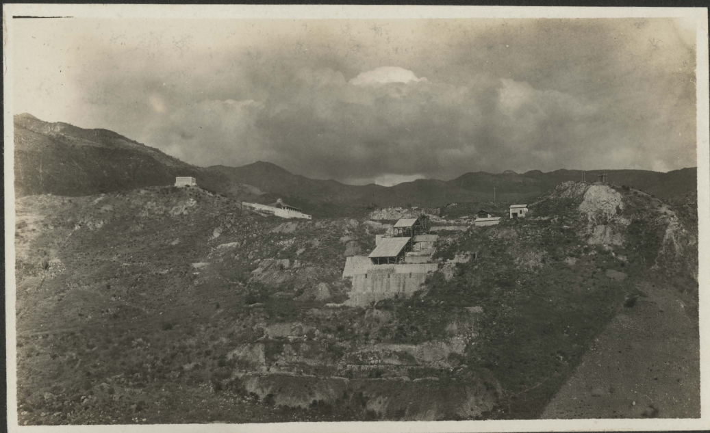
Mill building at Pueblo Viejo— (San Pedro Anasco.)
